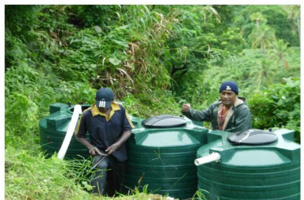
Villagers turn on the water
